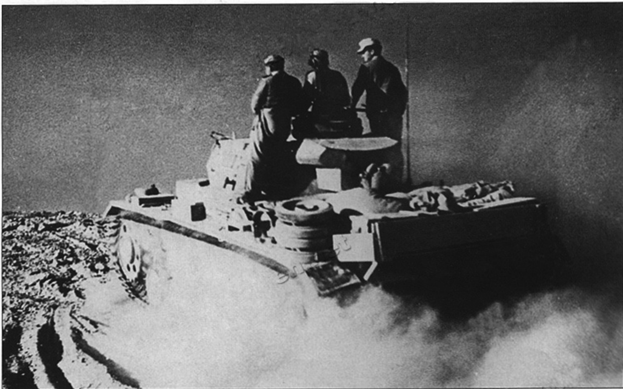
A lonely Pz.Kpfw. III kicks up a cloud of dust in the West African desert. A wooden storage rack has been added to its engine deck for easier transport of the crew's belongings. The tank is marked with large numbers, but only the first number is painted in red or black and outlined with white, which indicates the second company.
