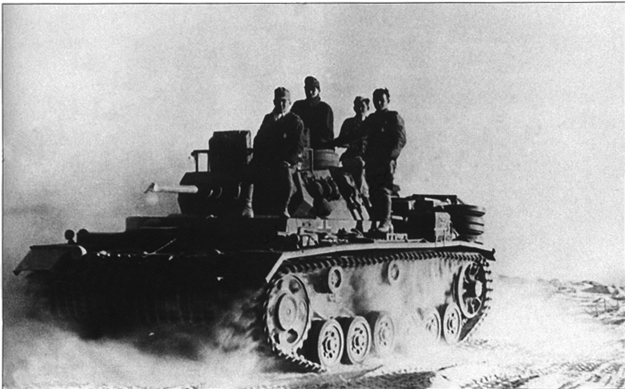
A Pz.Kpfw. III Ausf. J with a short 5cm gun stirs up the desert sand in February 1942. Note that the tank carries extra jerry cans and canteens on the turret, in the front of the command cupola, where a rack was installed to make their transport easier. This tank could be a remnant of the Balkan campaign.
