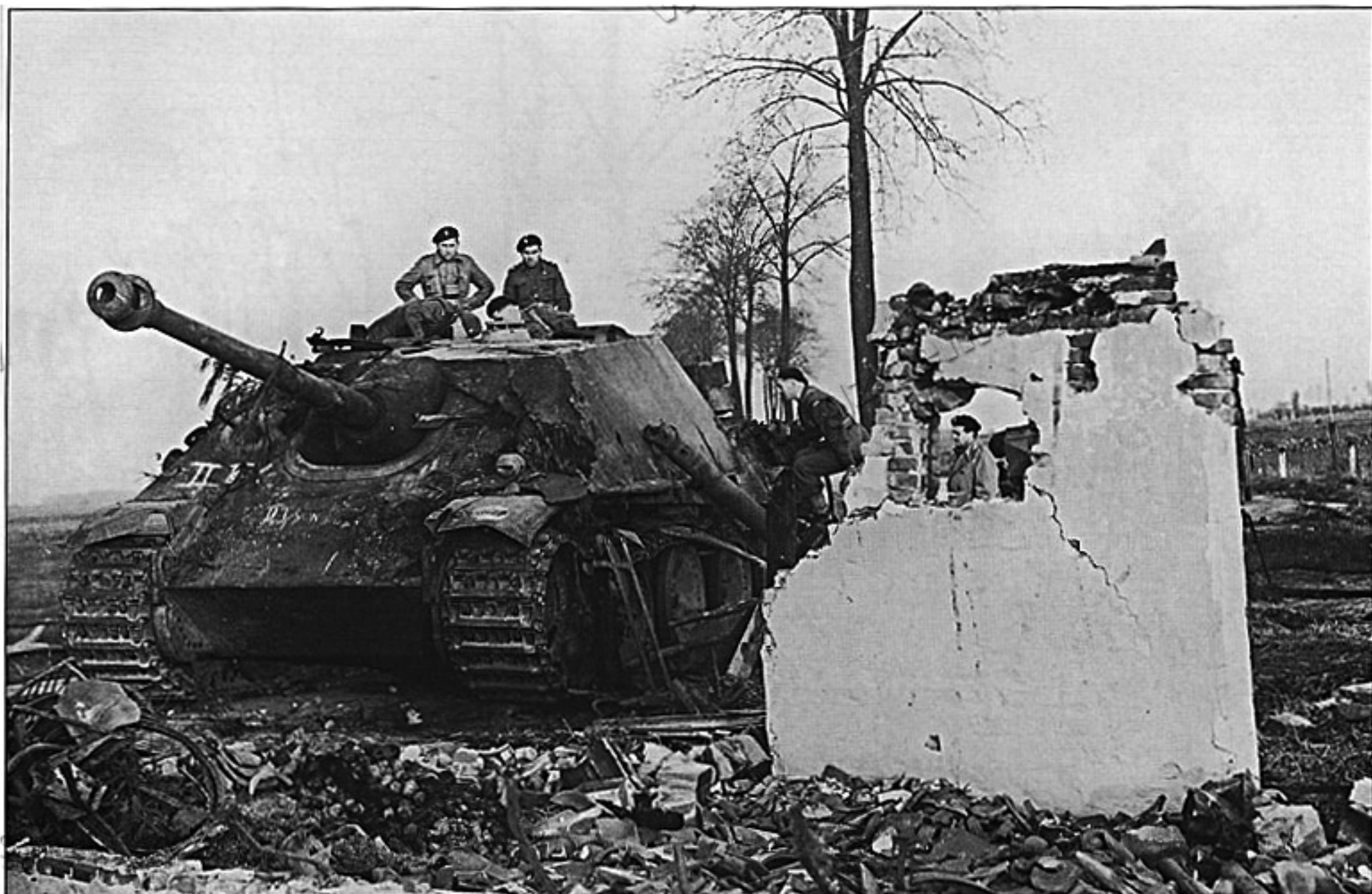
This Jäg.Pz. V "Jagdpanther" was knocked out of combat by the Polish 1st Armored Division at Langewes in Holland in late autumn of 1944. The vehicle burned up after it was hit in the side. The emblem painted on the right mudguard could be a German unit insignia. The Jäg.Pz. V was the best tank destroyer of its time due to its heavy weapon — the 8.8cm PAK 43 L/71 gun. It also benefited from very good armor protection that was designed in the Soviet style, which made this vehicle very similar to the tanks of the SU-122 family.
