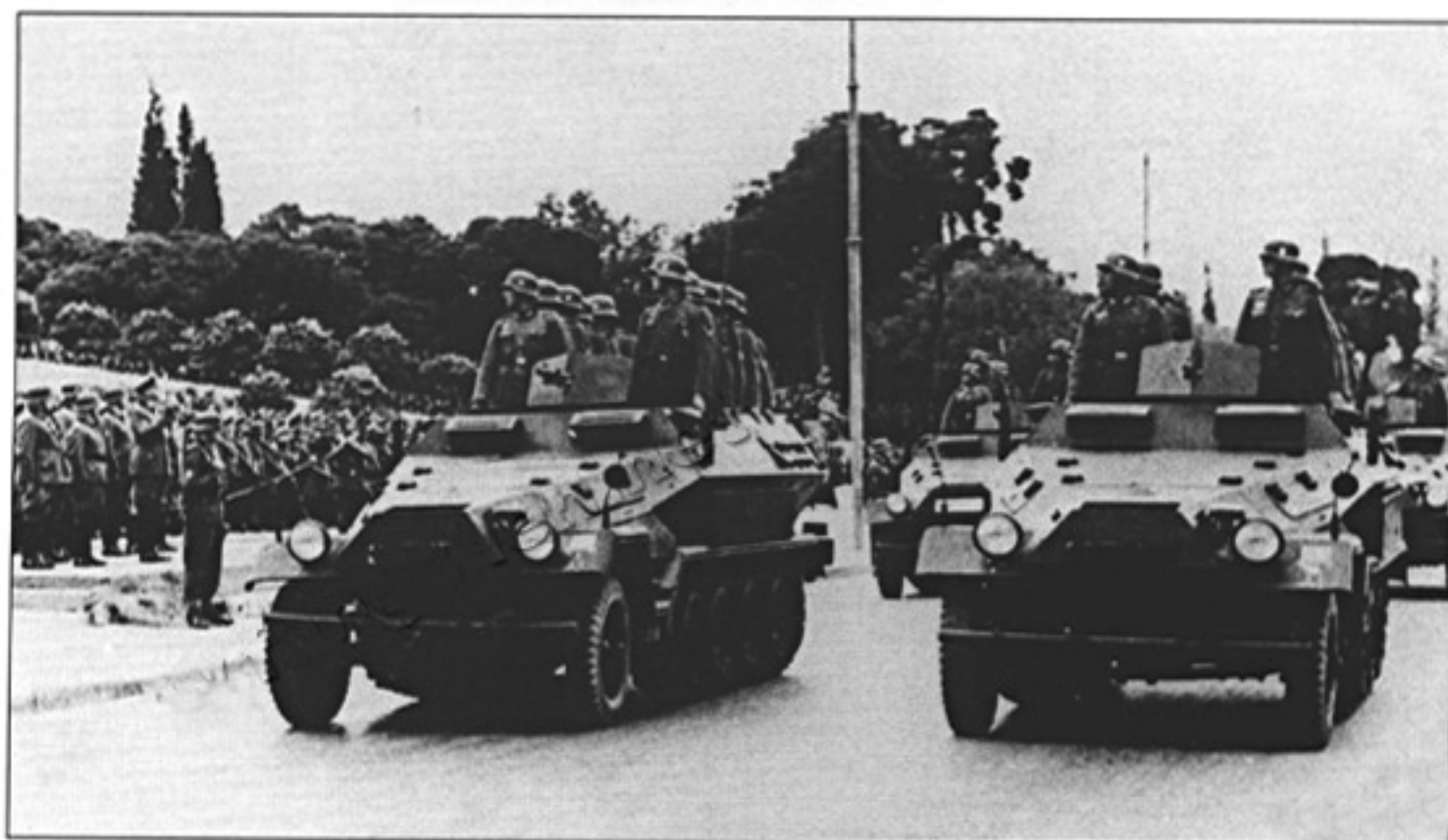
Following the conquest of Greece a victory parade was reviewed by Feldmarshall Wilhelm List in Athens on 7 May 1941. Note the tactical markings on the mudguards and the white national crosses barely visible on the side of the hulls of the Sd.Kfz. 251 Ausf. Bs.
