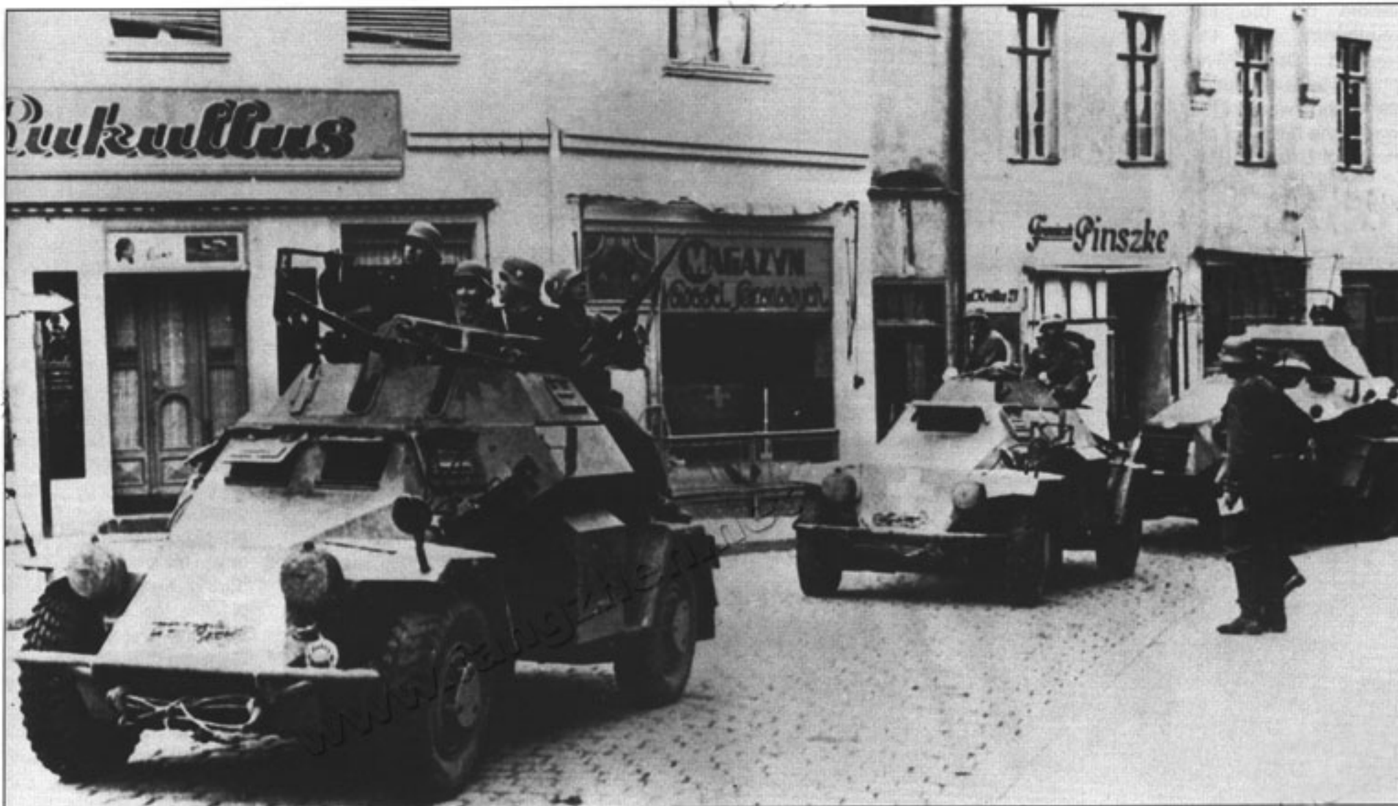
The lead armored cars of a reconnaissance unit from a Panzer division pass through a city in Poland. The first two vehicles are Sd.Kfz. 222s, the most popular German armored car of the whole war. Behind them may be seen a Sd.Kfz. 231, a three-axle heavy armored car first built in 1932. During the fighting in 1939 this AFV was judged to be obsolete, and its front line career slowly came to an end. Both leading cars have white crosses painted on the front plates, each being placed a bit differently. The second one has the same markings on the sides of its hull, as the reflection in the shop window attests.
