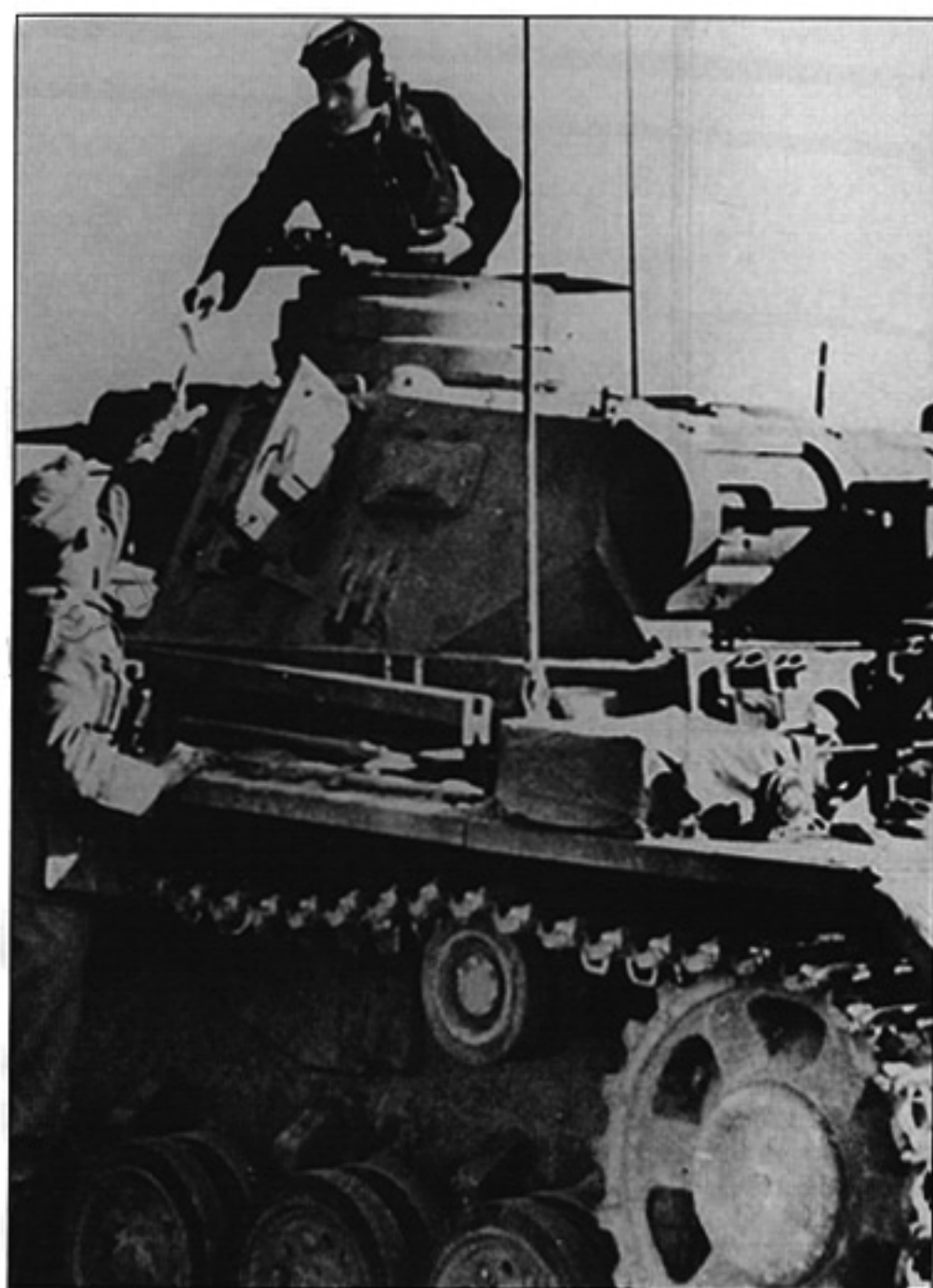
A staff officer in the cupola of a Pz.Bef.Wg. III Ausf. H from a Pz.Abt. belonging to 24.Panzer-Division relays some information to a soldier. Three antennae, including a frame antenna, are clearly visible. The vehicle is camouflaged with dark yellow paint, which was typical for German vehicles of this division on the Eastern Front in June-July 1942. It also carries a small white tactical number "110", which is partially obscured by camouflage. Note the additional armor plate installed on the front of the superstructure.
