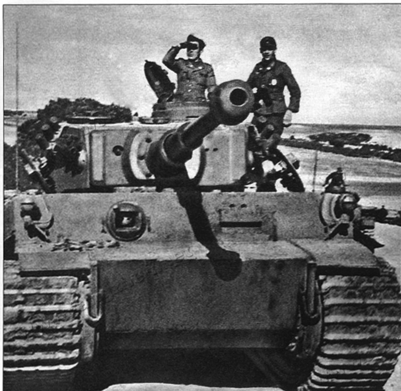
This Pz.Kpfw. VI Ausf. E of sPz.Abt.501 was photographed just after its arrival in Tunis in February 1943. The tank shows the typical sand brown color worn by the tanks in this unit. Some vehicles were painted light olive green in the spring of 1943 to match the grassy hills of Tunisia. Note the unit's elaborate field modification of placing the Bosch headlights in a new position on the front plate of the superstructure.
