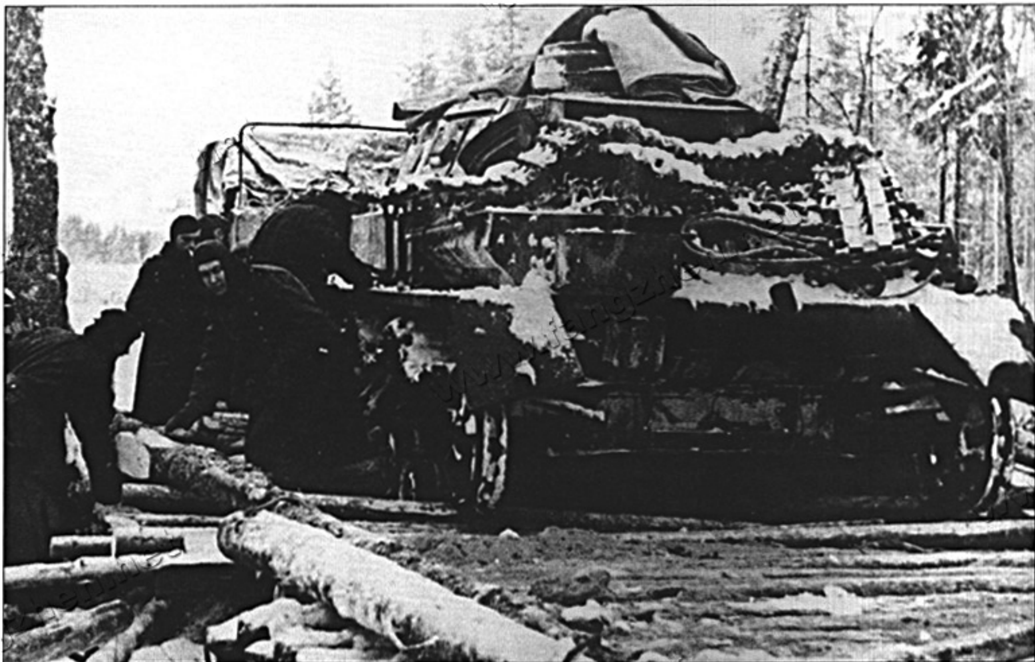
Another recovery mission, this time accomplished by a heavy tractor in difficult forest terrain. The Germans tried to tow the Pz.Kpfw. IV on a specially prepared platform built of logs, but some of them were too weak and broke under the weight of the tank, blocking the last two road-wheels. Many similarly damaged tanks were abandoned by the Germans during the great winter retreat of 1941/42 due to a lack of fuel, tractors and time.
