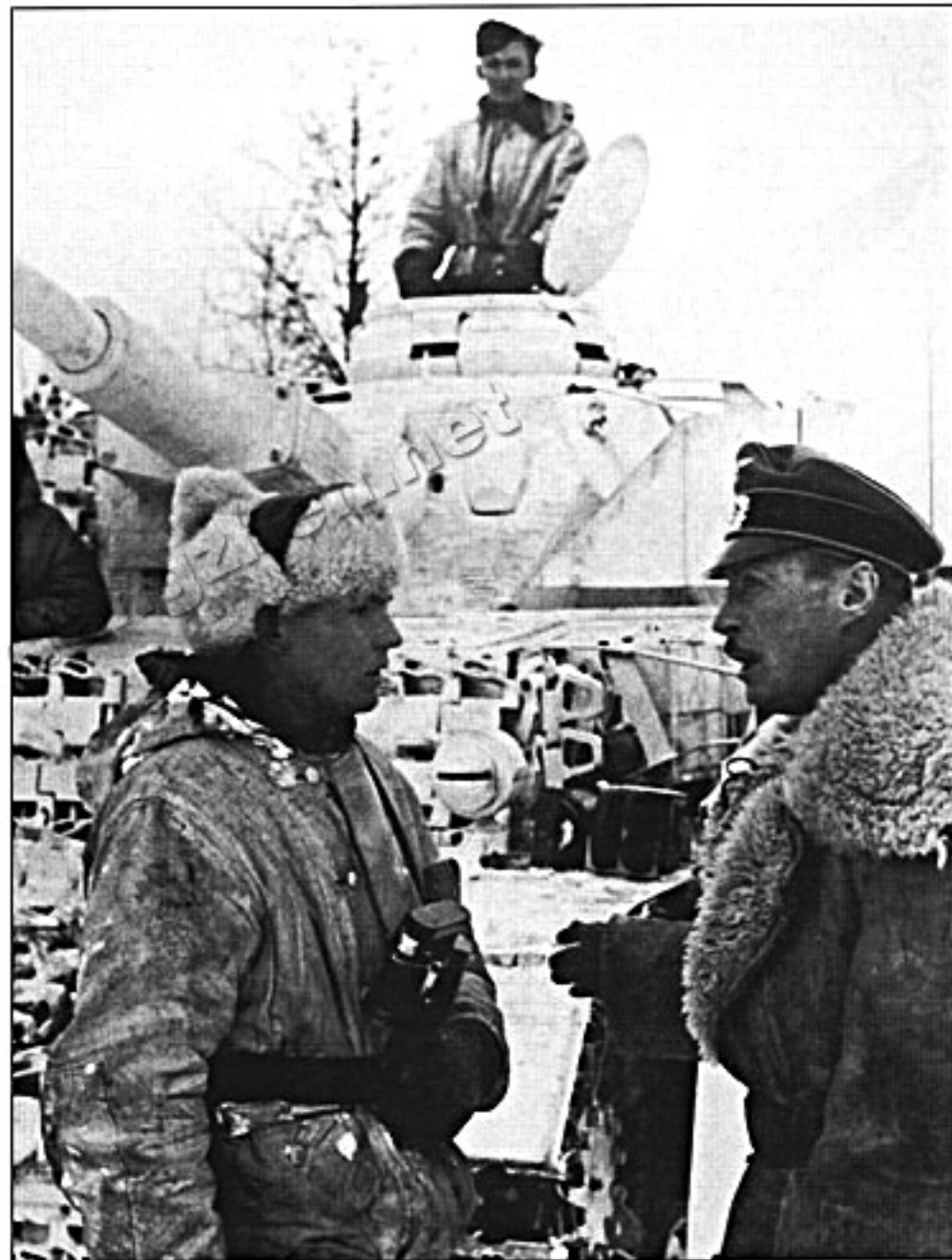
Generalmajor Graf Strachwitz is seen inspecting a StuG unit at the Narva front. The StuG III Ausf. G seen in the background carries a heavy coat of white camouflage painted with care by spray gun. Note the wooden box installed next to the machine gun shield, very untypical for the StuGs. Of special interest is the unit emblem painted next to the gun mantlet.
